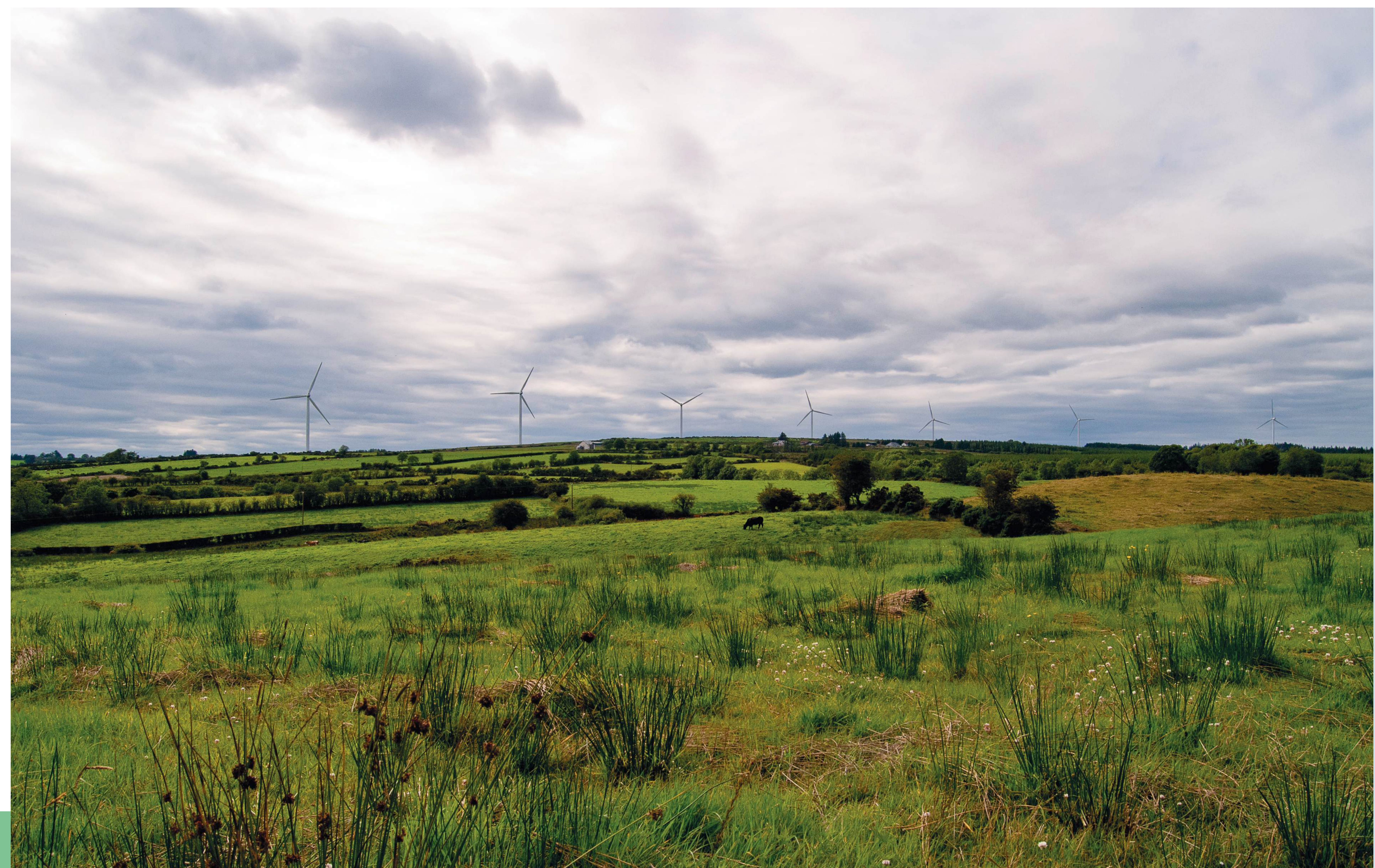
Glenough wind farm
