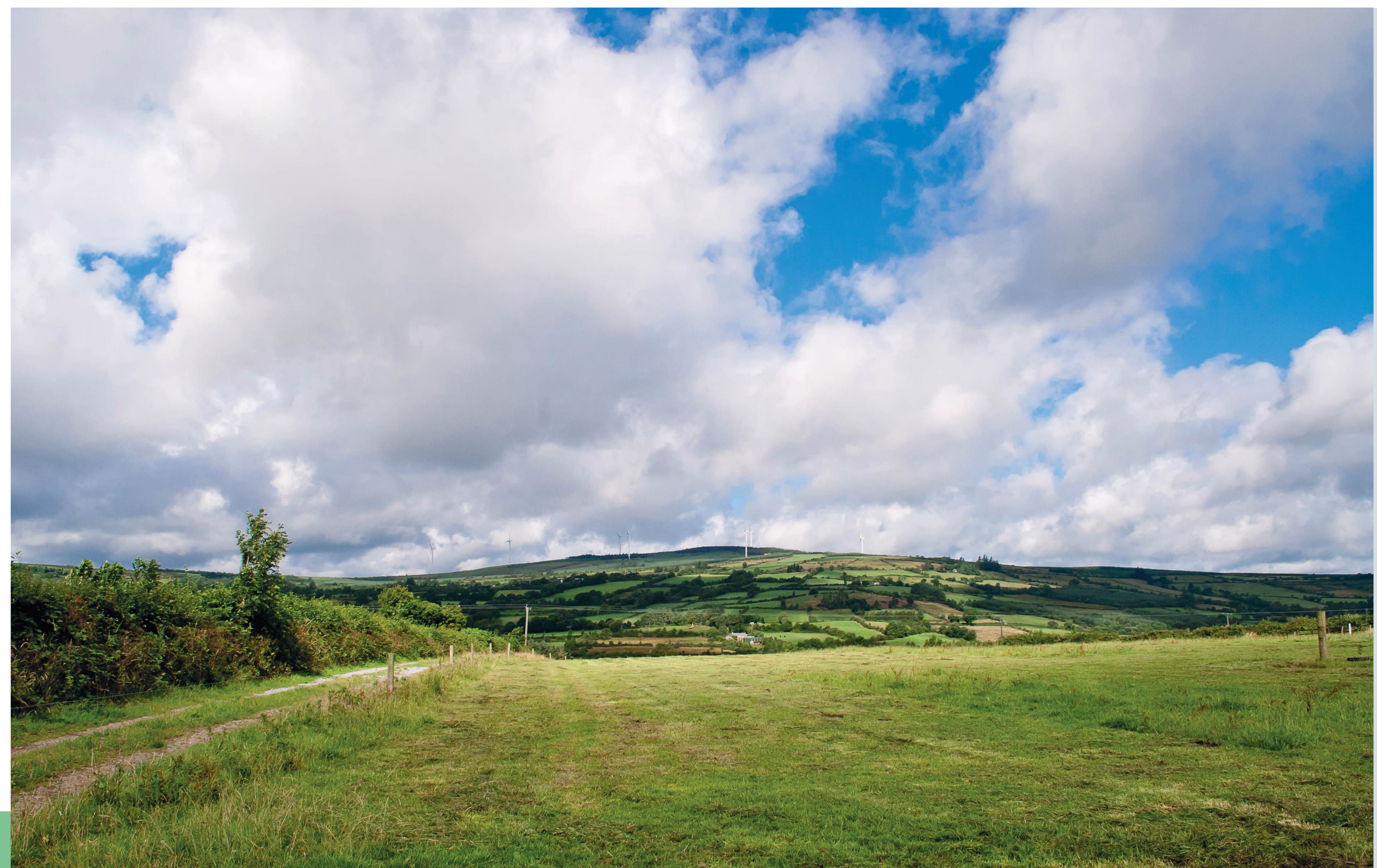
Glenough wind farm
